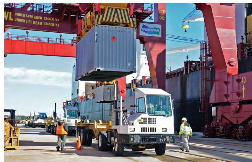
ABOVE: Stevedores guide a container from the crane's spreader bar onto a "bomb cart" trailer during a cargo offload using new ship-to-shore container cranes at the recently renovated center wharf at Military Ocean Terminal Sunny Point, North Carolina.
