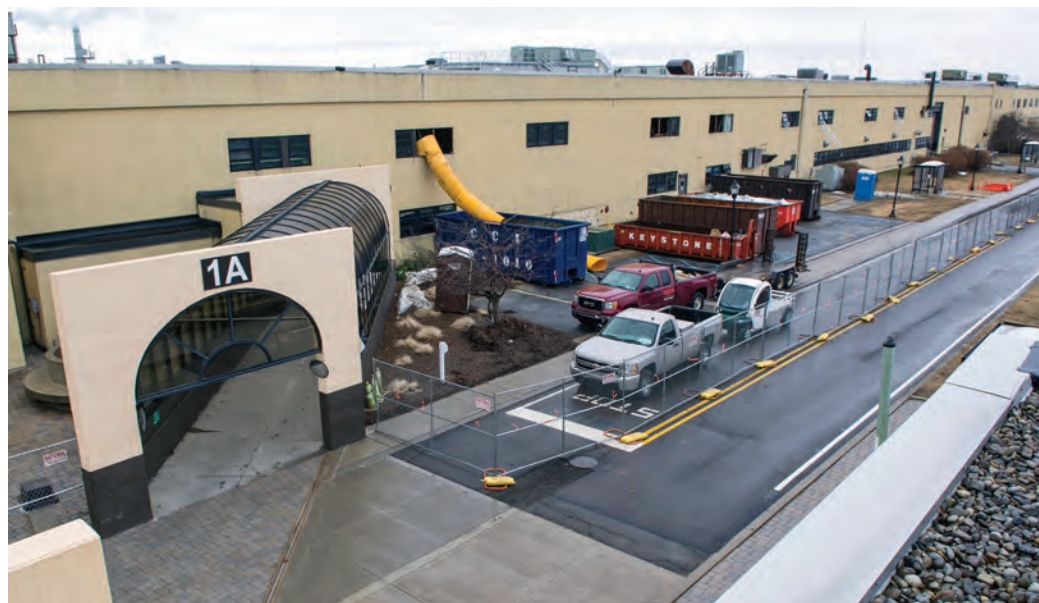
LEFT: Tobyhanna is undergoing a massive, multiyear effort to upgrade facilities. The $102 million investment includes everything from replacing thousands of lights to updating nearly 200,000 square feet of industrial and engineering space in the heart of the electronics maintenance complex. (U.S. Army photo by Steve Grzedzinski)
