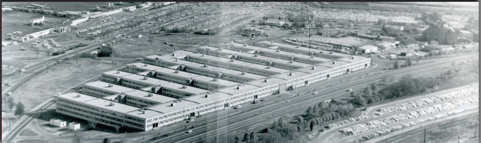
Above: AMC Headquarters, Building T-7 adjoining National Airport
