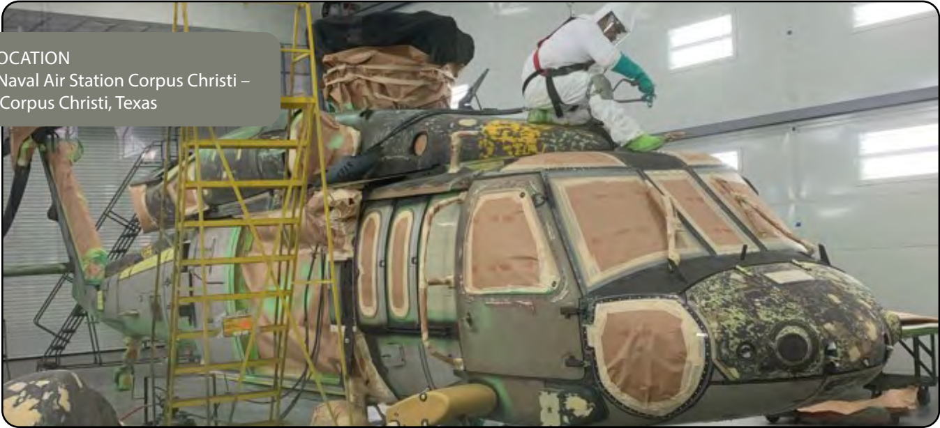
A Corpus Christi Army Depot painter journeyman applies the new "Class N" primer undercoat to the first Army Black Hawk helicopter. The process removes heavy metals from primer operations during aircraft maintenance. CCAD leads the way in implementing controls and protections for safer environments in depots and in the field where Soldiers and civilians perform maintenance. (Courtesy photo)
